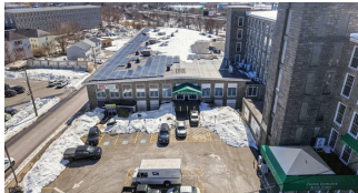
Tower Mill Self Storage
